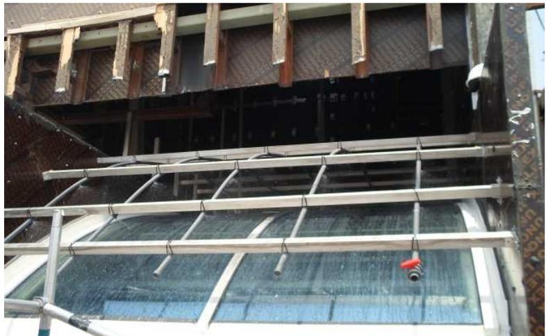
as per Qatar Construction Standards. Two types of steel frames have been designed, one to support both the glazing and aluminum sandwich panels, and another to transfer all the loads to the main structure.
